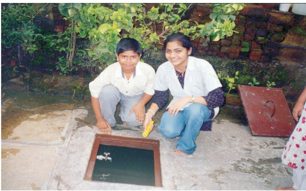
Fig. 2. Inspecting underground water storage tank
